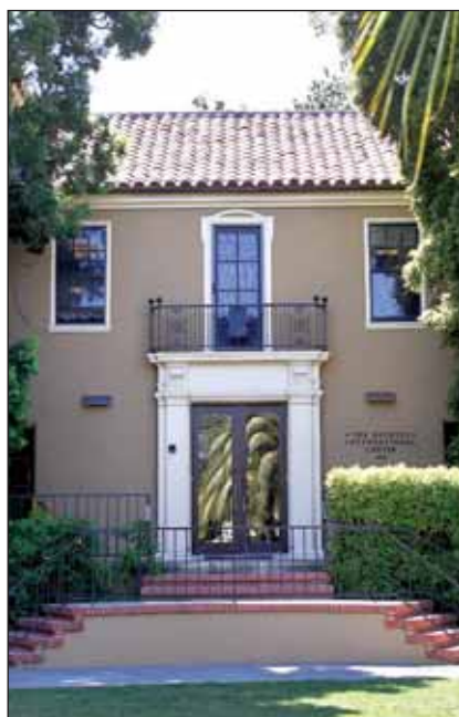
Inset Moorish arches, middle, are an unusual touch to the Spanish Eclectic Bechtel International Center, featured on the Stanford Historic Houses walking tour. The Bechtel International Center, above, designed by architect John Branner in 1917, will be featured on the Hidden Gems of Upper Lomita tour at Stanford University.
